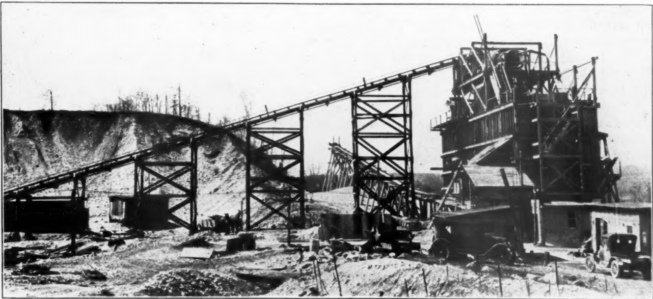
The Main Screening and Storage Unit is the Building at the Right
